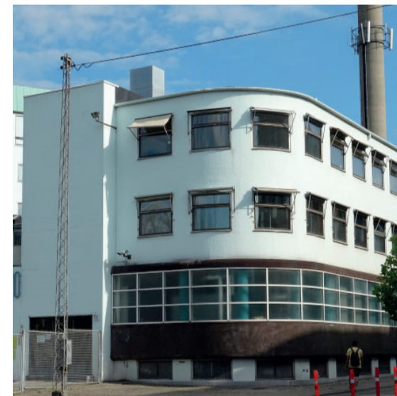
Novo fabrik, Arne Jacobsen, 1933 - 1969
