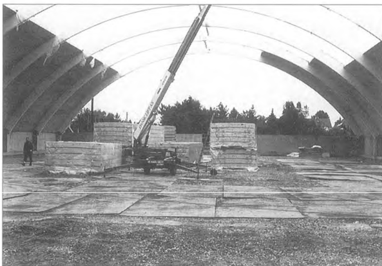
Ny tennishal under opbygning, 1993.
